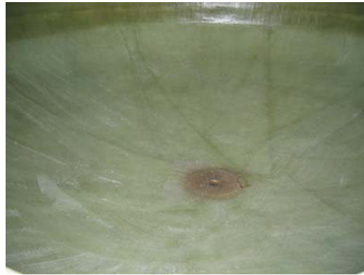
Figure 9.2: Storage tank with a curved bottom and without inside frames making drainage easy (Photo: Bjørn Løfsgaard)
