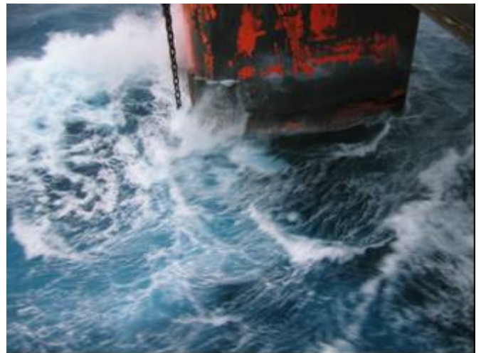
Figure 6.1: Normally there is great turbulence in the water around the platform legs and the sea water intakes should be placed where the danger of pollution is at a minimum (Photo: Eyvind Andersen)
