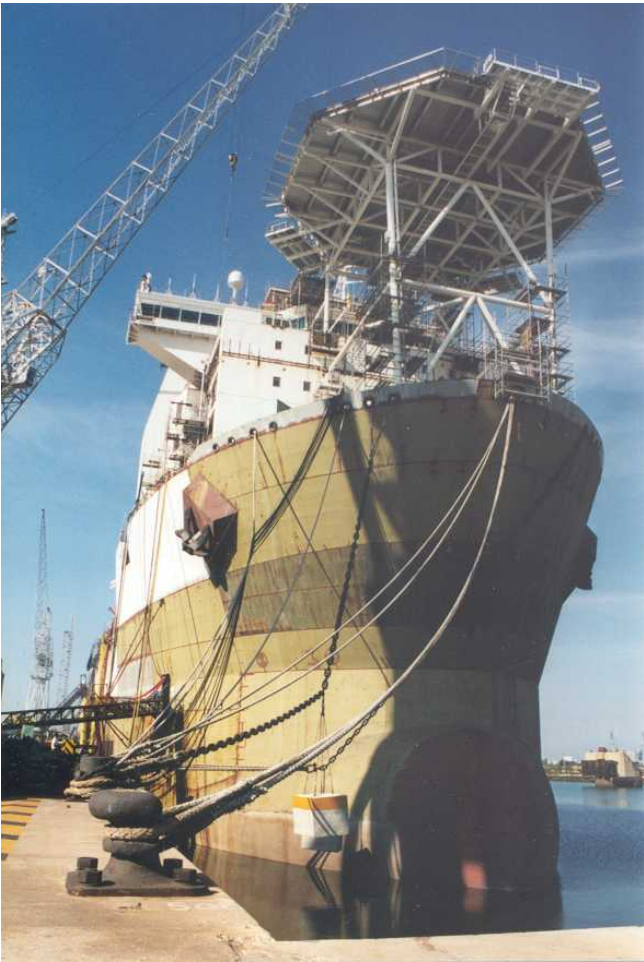
Figure 2.1: Picture taken at the shipyard of the Navion Odin unit (Photo: Eyvind Andersen)
