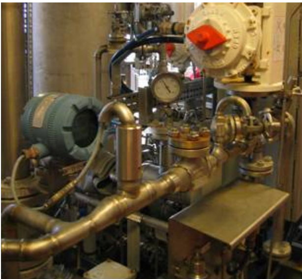
Figure 6.7: A conductivity meter automatically measures salt content in produced water and dumps it if the 6 mS/m limit is exceeded (Photo: Eyvind Andersen)
