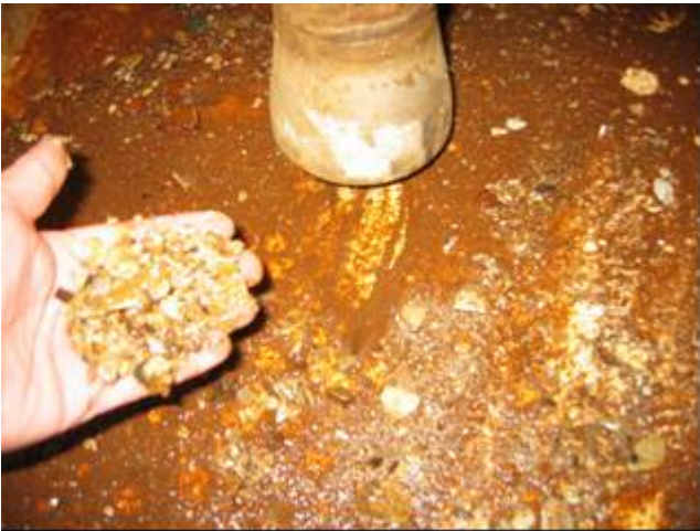
Figure 8.4: In unstable weather particles and sediments in the potable water tanks can be whirled up and sucked into the distribution system, reducing the effect of the UV radiation. (Photo: Bjørn Løfsgaard)
