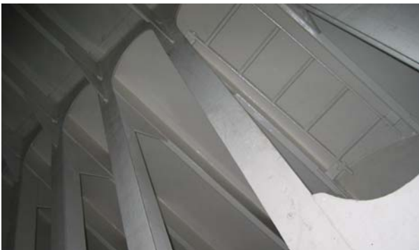
Figure 9.4: Picture of a storage tank with newly applied protective coating. In a tank with a large inner surface compared to volume, the risk for growth of micro-organisms increases, as well as problems with unpleasant smell and taste (Photo: Eyvind Andersen)
